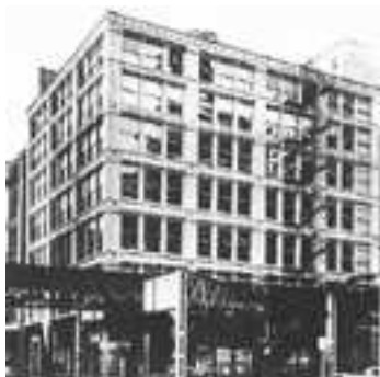
Foto 11 – First Leiter Building : fachada
