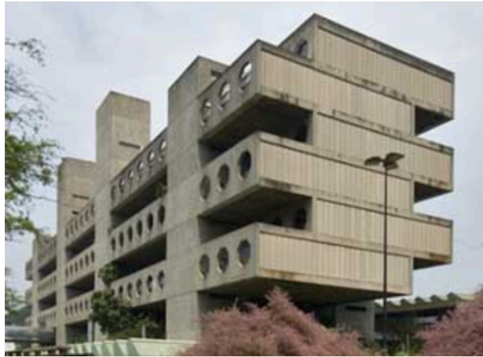
Figura 11 - Hospital Sarah fachada lateral
