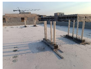
Figura 11: Bases nos tubos
